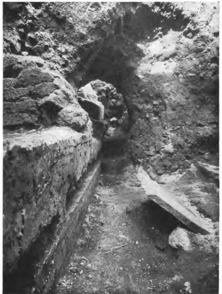
Fig. 111 — S. Lorenzo f.l.m. Basilica maior , dig 5, foundation wall of colonnade, from west (Photo: Sansaini).
